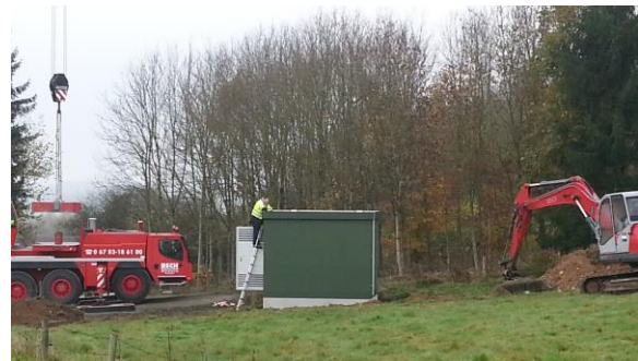
Interconnection work at Wind Works Elkfarm 1
