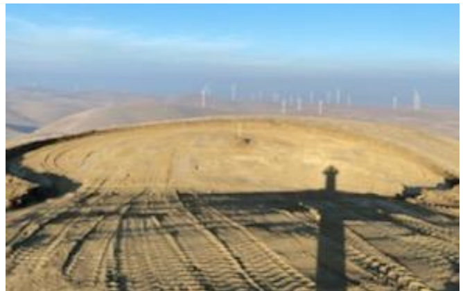
Start of construction in the US with foundation excavation.
