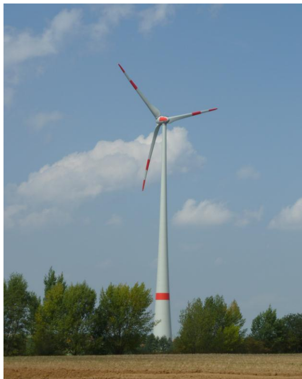
Wind Works Project Burg 1 in Operation
